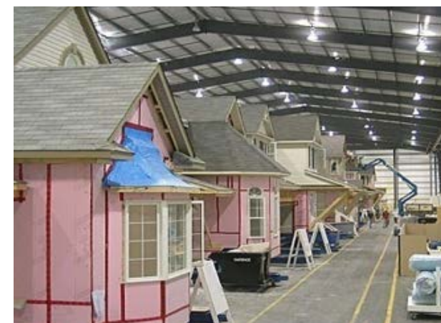
Caption: Continuous Flow Production Technique of Knock-Down House
