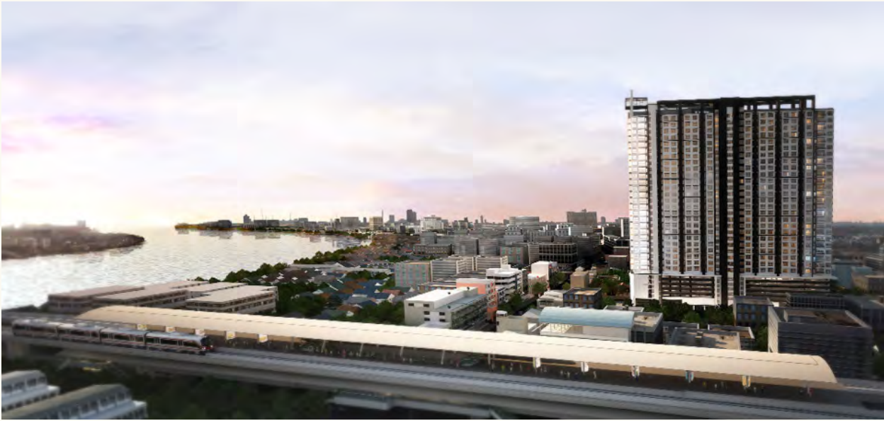
The Tree Bang Po Station Project
