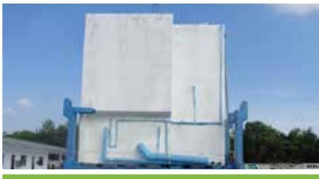
Transport Rack Bathroom Pod
