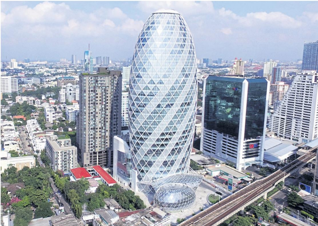
The 3-billion-baht Pearl Bangkok, a 25-storey LEED-certified green building at gold level, is owned by Thongma Vijitpongpun, group chief executive of Pruksa Holding Plc.
